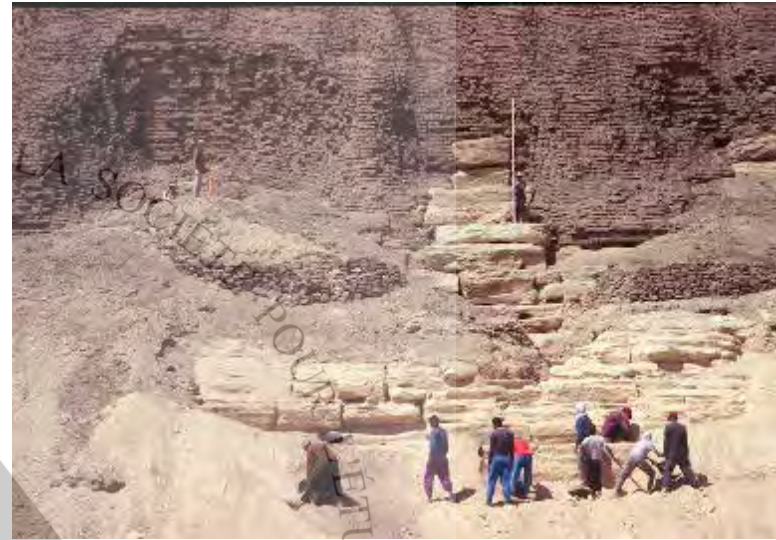
Figure 3-60 – View of Upper sub-casing blocks with Axial Cross Wall above (JEK and RAF surveying).
