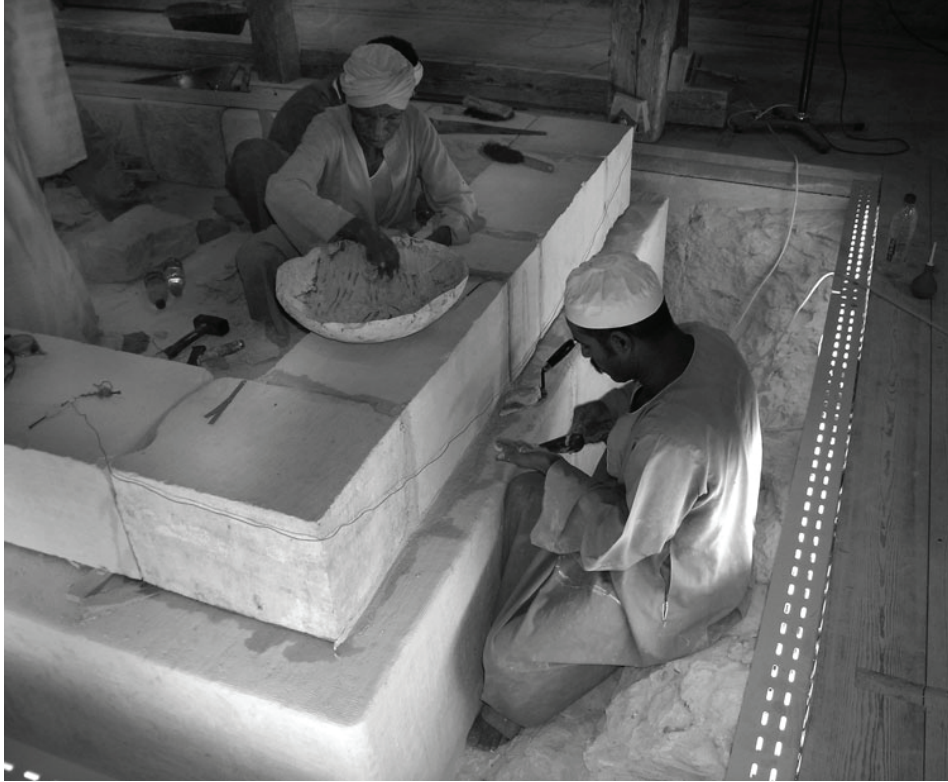
Figure 5: Workmen rebuilding base of sarcophagus box on top of calcite plinth
