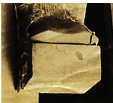
Figure 10: Stanford Museum: detail of staining on pedestal in Figure 8; Stanford Historical Photograph Collection, SHPC ID 6273.
