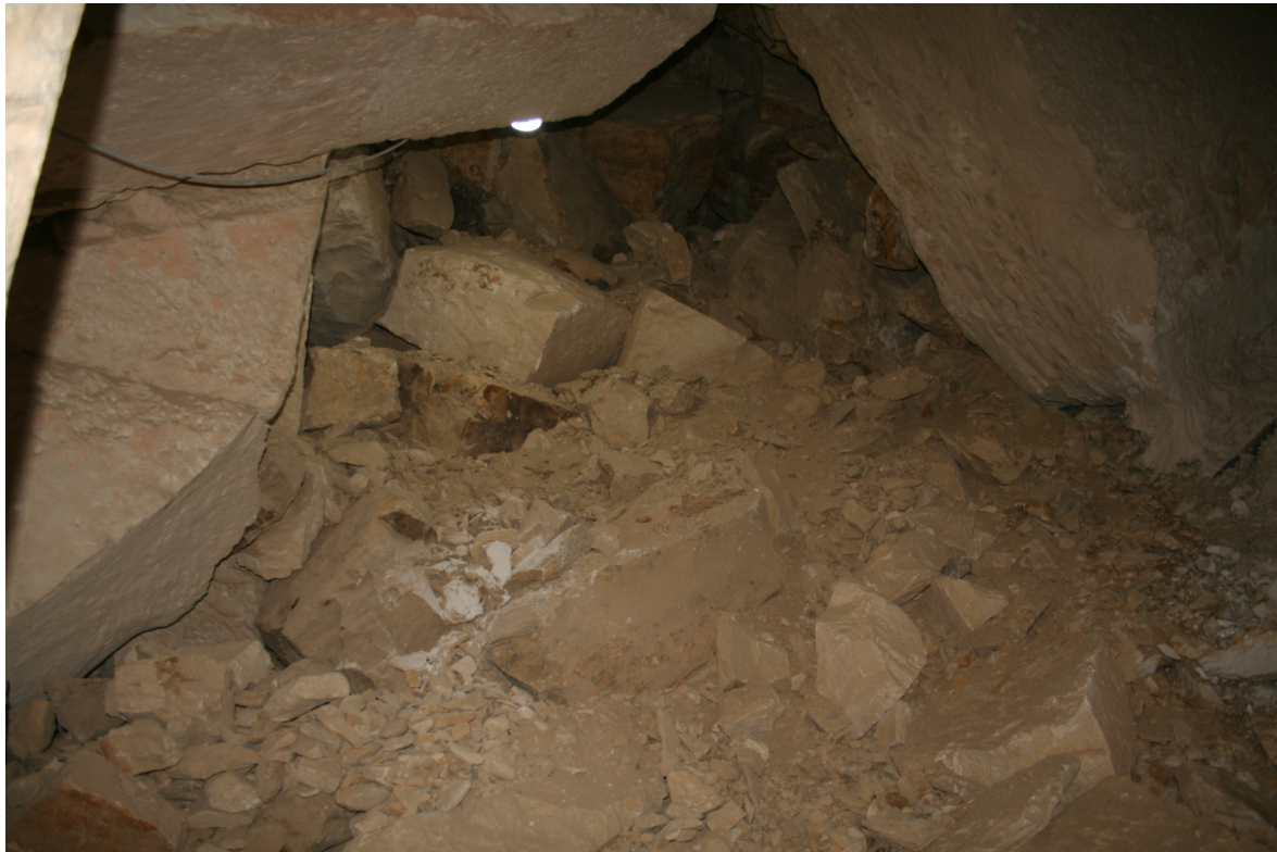
Figure 11. The falling blocks from the eastern side of the pyramid into the antechamber. (© Abusir Project, photo by M. I. Khaled).
