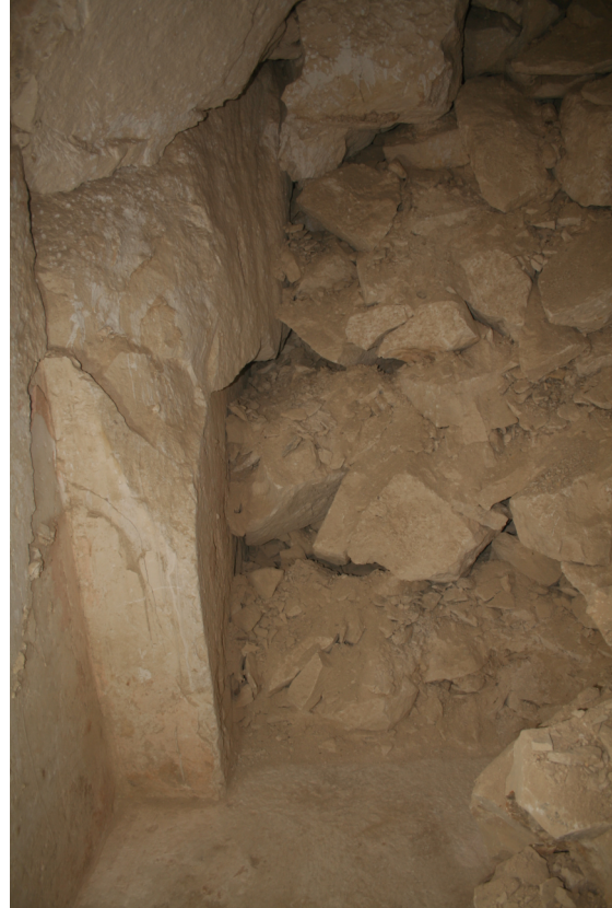
Figure 12. The northern wall of passage with the remains of its ceiling. (© Abusir Project, photo by M. I. Khaled).
